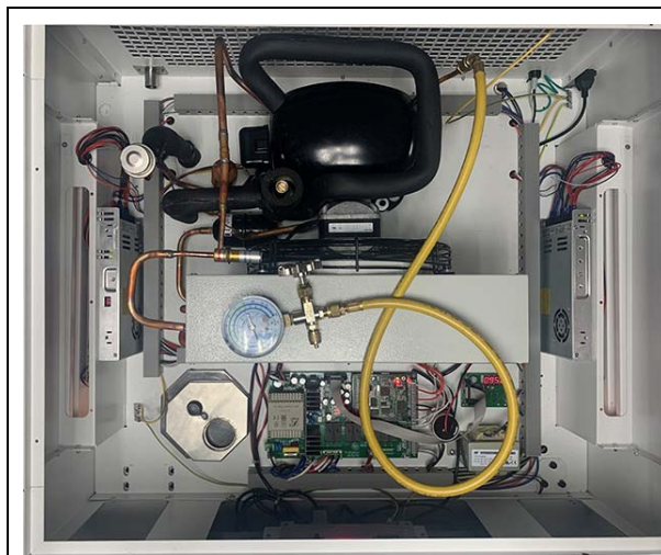
Fig 43 Checking and charging of the refrigerant
