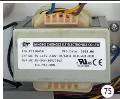
70 Ultra-sonic generator for piezoelectric elements 75 Power transformer
